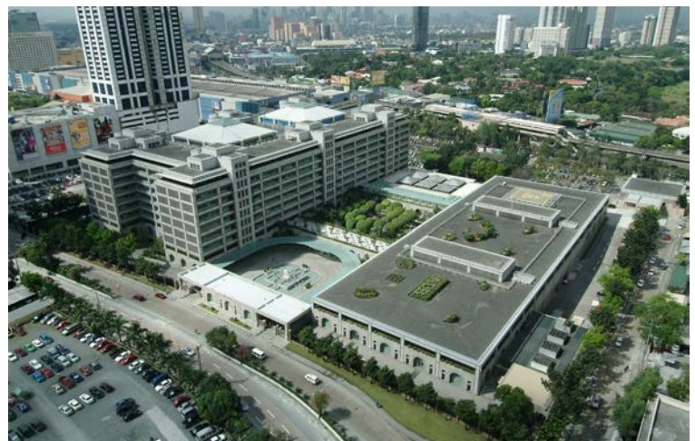
Asian Development Bank Headquarter Source: ADB, 2013
