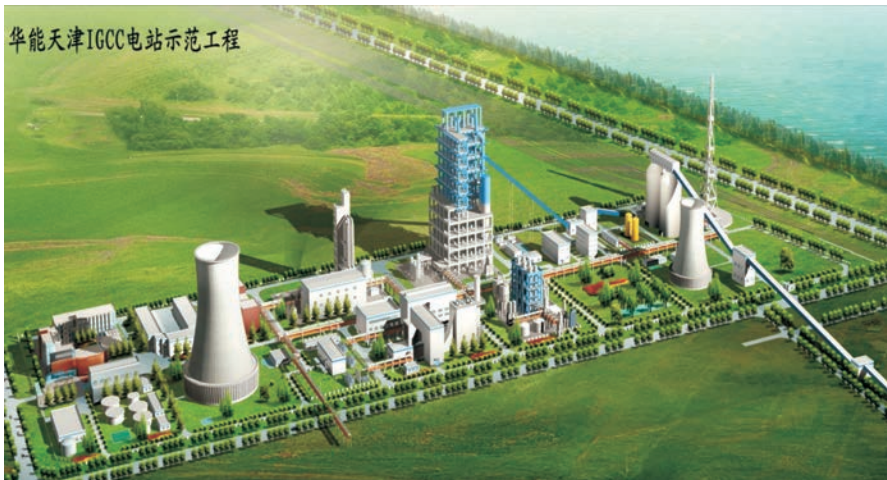
Tianjin IGCC Power Plant
