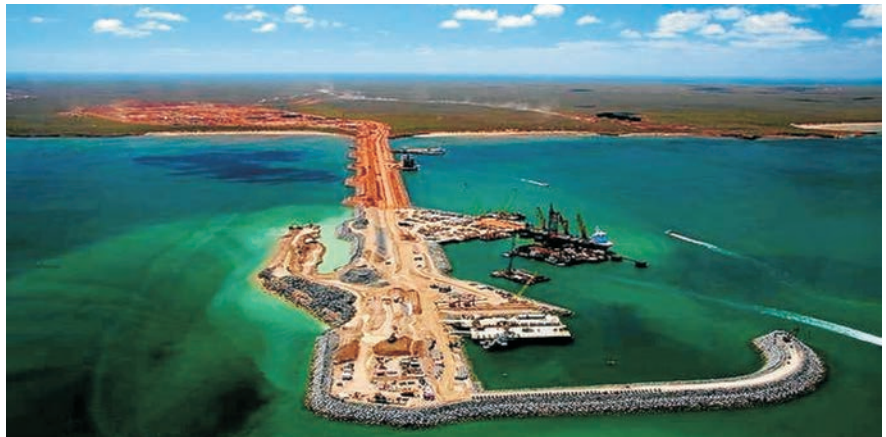
Gorgon LNG Terminal in Construction, Barrow Island, Australia
