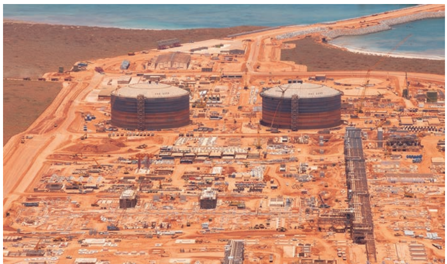
Gorgon Project in Construction
