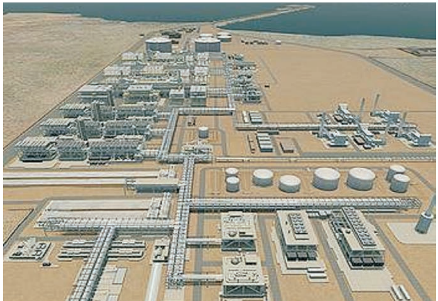
Australia Gorgon Project Gas Processing and LNG Terminal Montage
