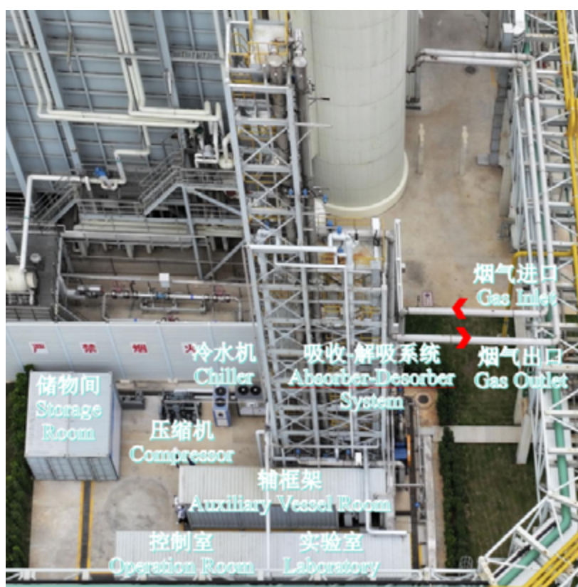
Fig. 13 Testing Platform Equipment Layout
