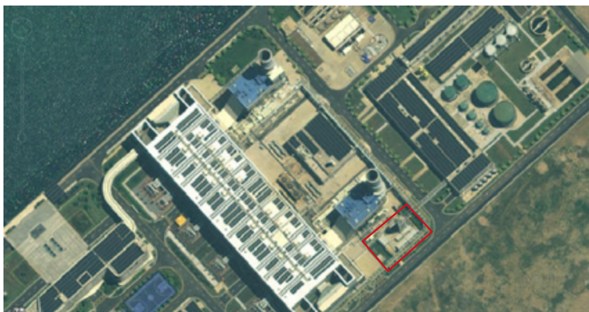
Fig. 8 General layout of Huaneng Yangpu NGCC plant, showing the location of the CO 2 capture platform (red highlighted area). The platform was designed in conjunction with the power plant.
